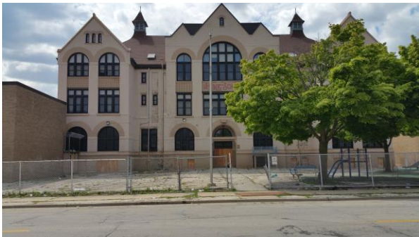
Garfield (July 2015) – Unused MPS building
